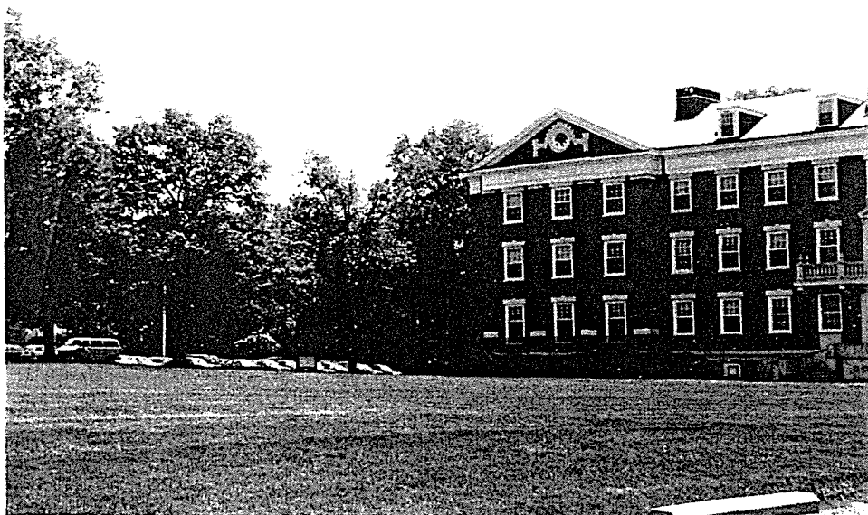
PHOTO ID: Building 007 and Lawn Panel, looking south, 5/97
