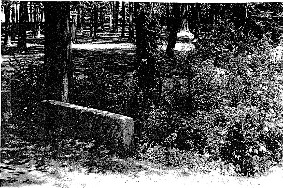
PHOTO ID: Drainage channel at 2nd St. near picnic grounds and residences, looking northeast, 5/97
