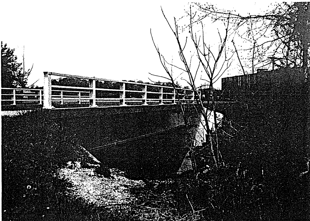
PHOTO ID: Bridge, looking east, 4/97
