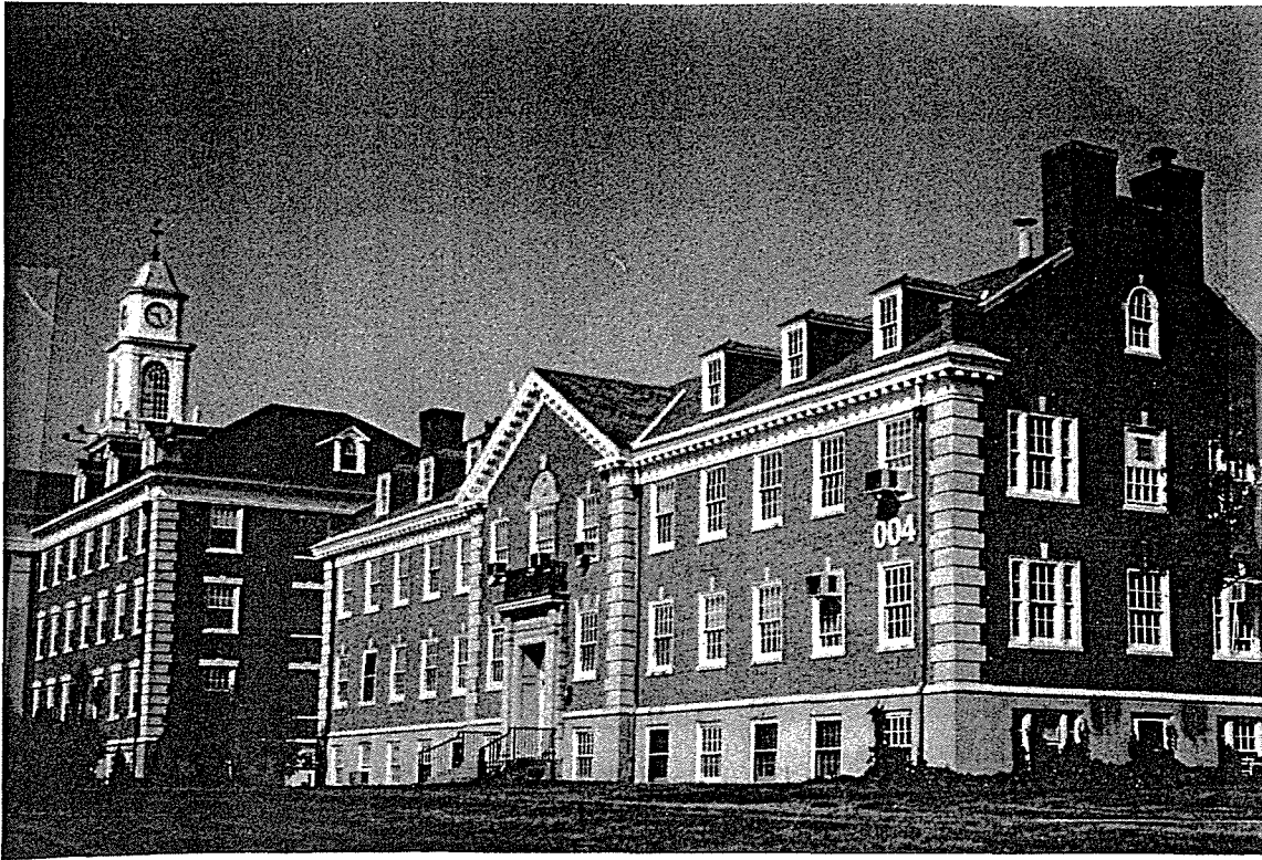
PHOTO ID: East facade of building 004, 5/97
