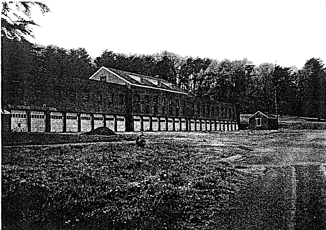
PHOTO ID: South Farm Service Road/Building 060/Fire Hydrant, looking west, 4/97
